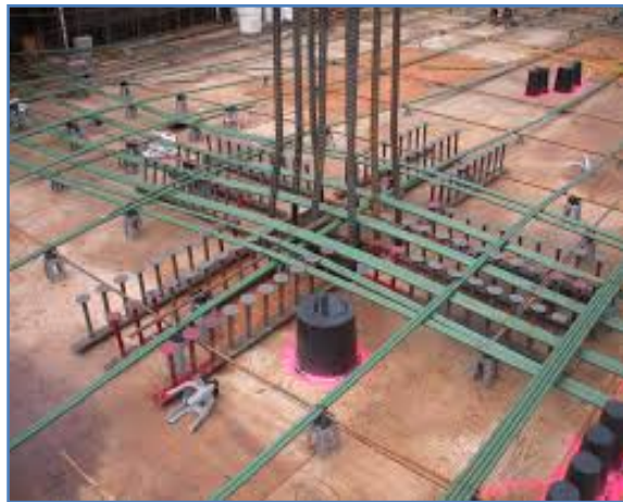
Figure 8. Unbonded Post Tensioned Slab
